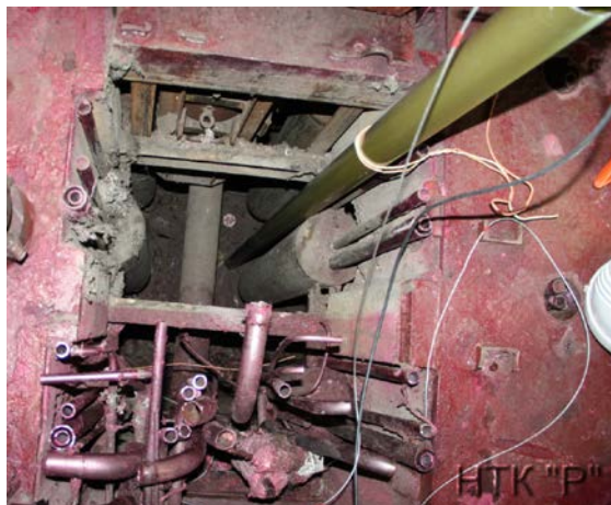
Fig.4. Container with radioactive ion-exchange resins and aluminum tube.
